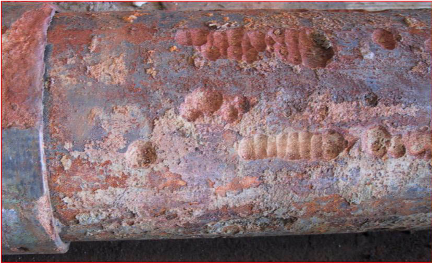
Tong marks with corrosion
