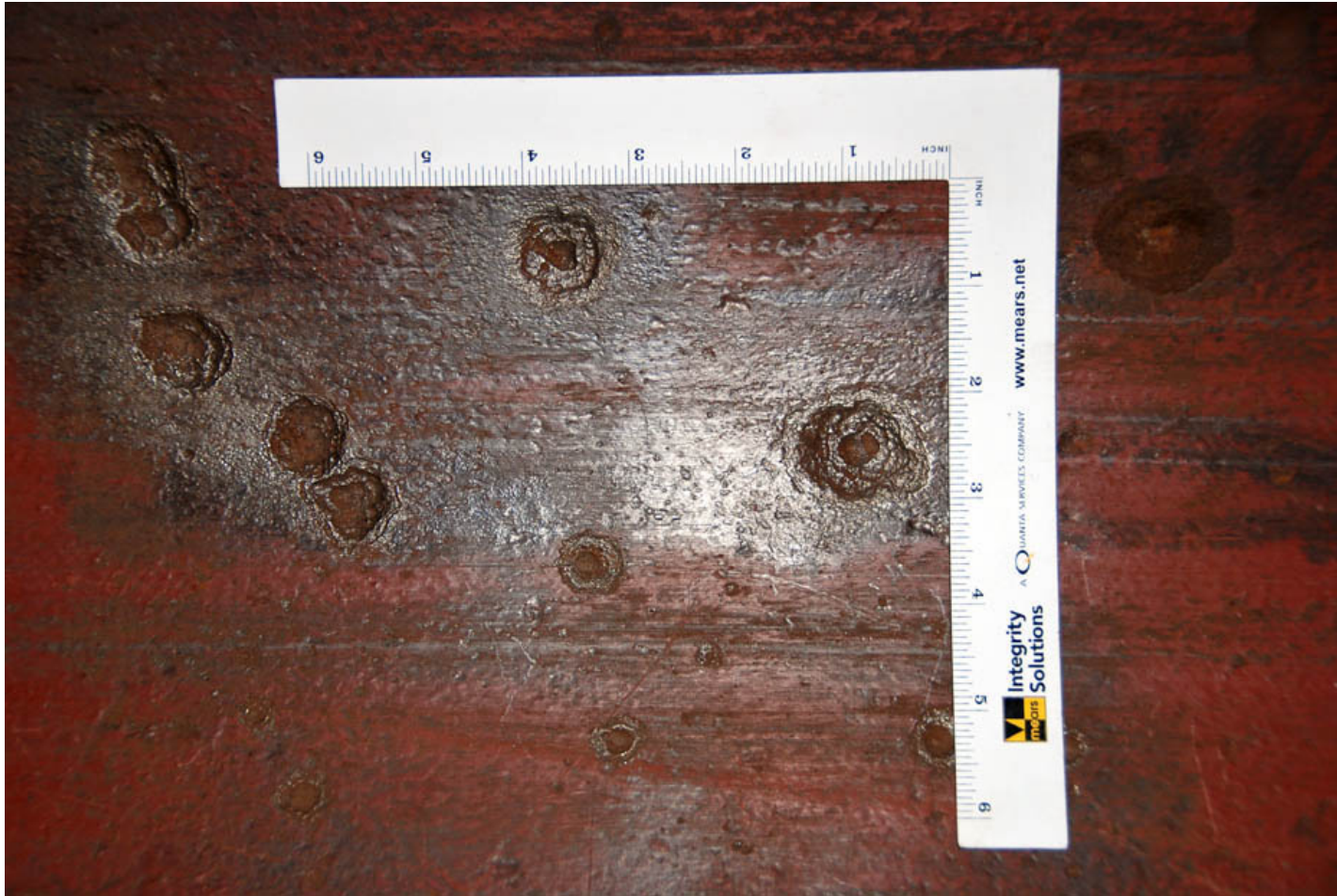
SRB (Sulfate Reducing Bacteria) Corrosion
